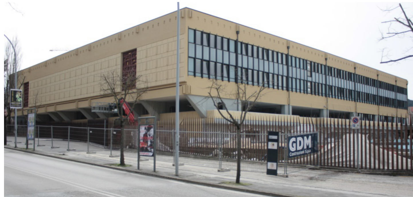
Above. Court of Law in L'Aquila. The building has been heavily damaged during the 2009 earthquake.
